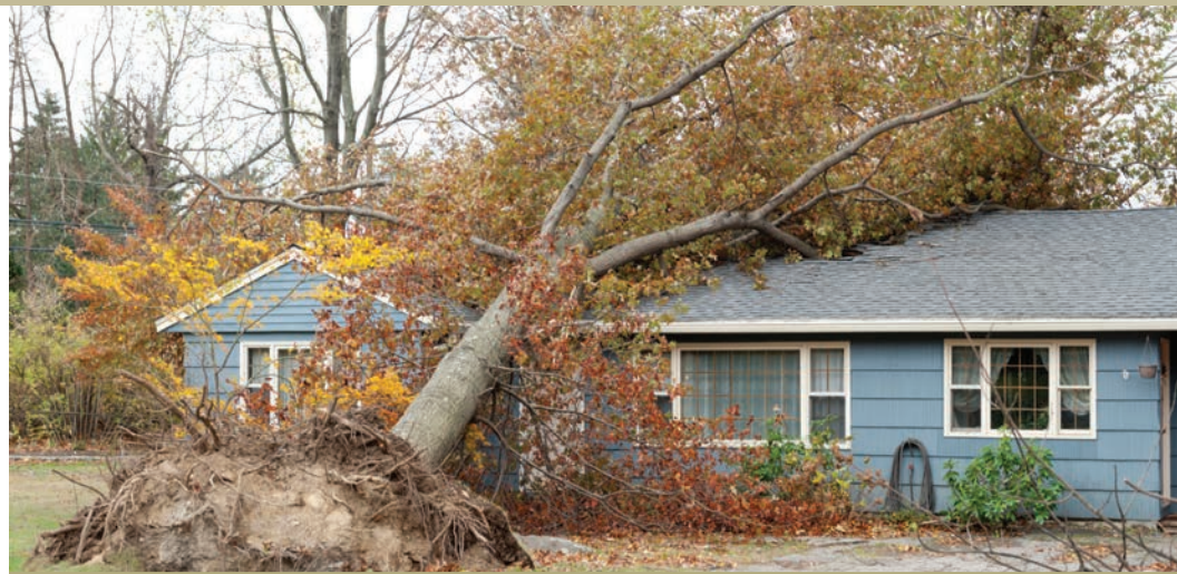
Damage caused by Hurricane Sandy in Connecticut
