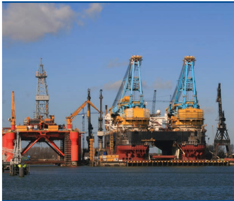
Oil drilling platform under construction on the North Sea
