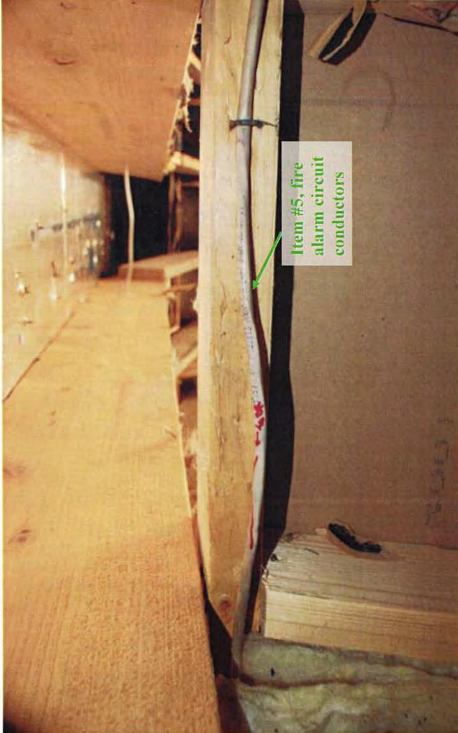
Photograph 12: View of the position along the northern living room wall where the fire alarm circuit conductors (item #5) were cut for removal at the field-applied red marking.
