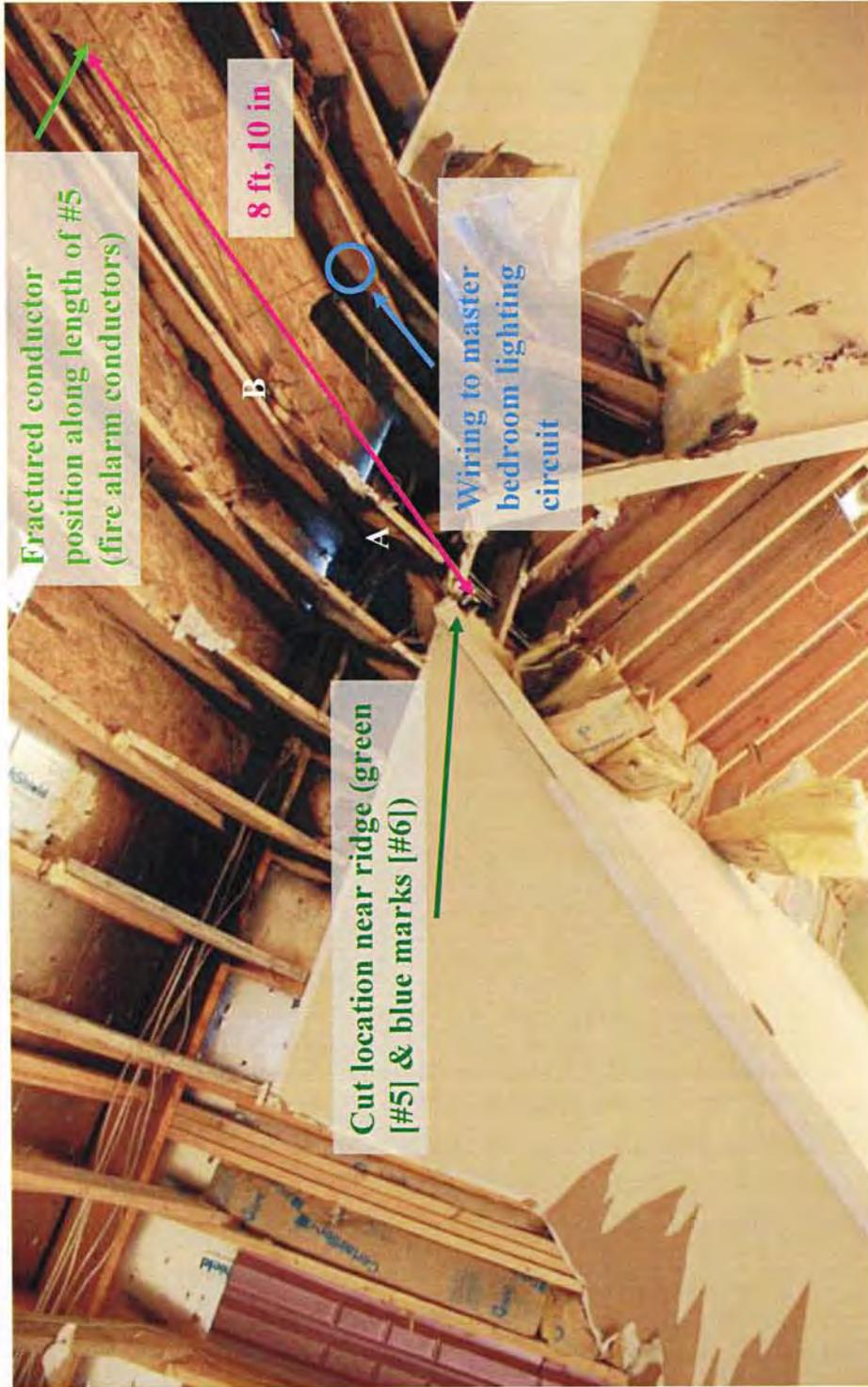
Photograph 3: Alternative view of the living room ceiling/attic space. Artifacts of electrical activity on item #5 identified during my October 21, 2011, field inspection were positioned upslope from and outside of the area of fire origin described in my original report.
